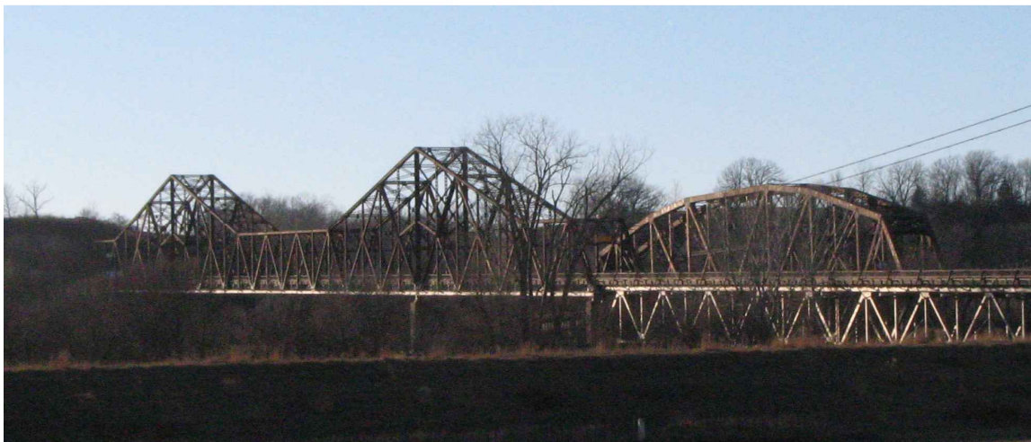
Figure 2-2. Plattsmouth Bridge over the Missouri River connecting Nebraska to Iowa built in 1929 (Image credit: http://www.wikipedia.org/ )
