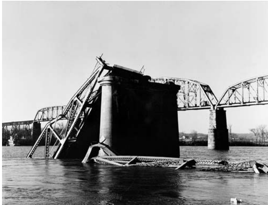
Figure 2-3. Silver Bridge failure over the Ohio River caused the death of 46 people in 1967 (Image credit: http://www.pbs.org/ )
