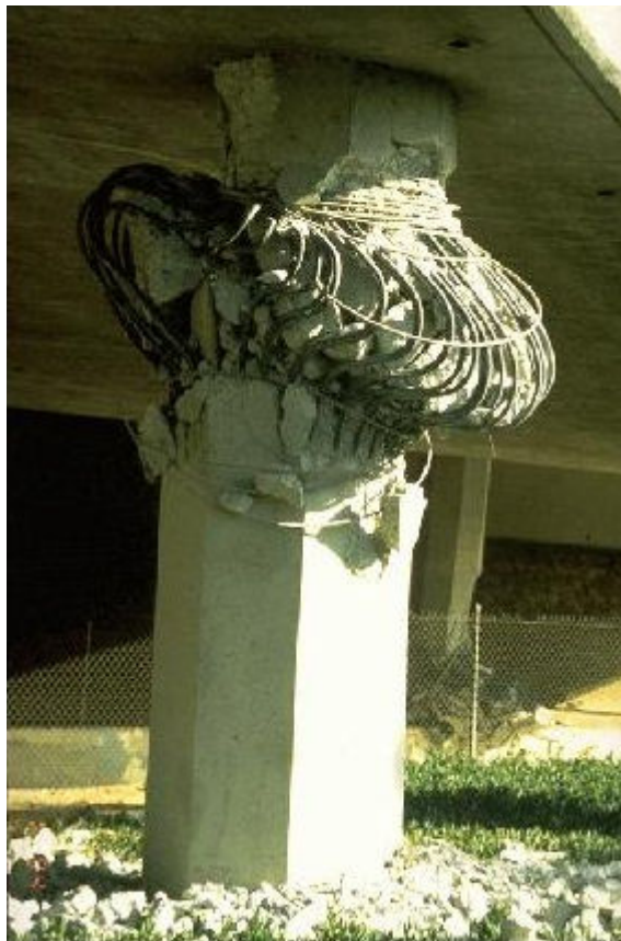
Figure 3-1. Plastic deformation of a bridge concrete column during the 1994 Northridge earthquake (Image Credit: NOAA/NGDC, M. Celebi, U.S. Geological Survey)
